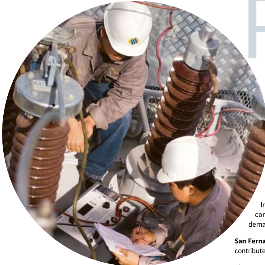
Subic EnerZone personnel test equipment at the Cubi Point substation.
